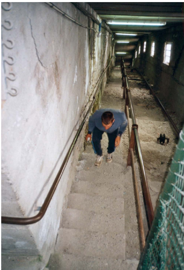
Fig. 2. The covered stairs at the Turin hut. The participant will arrive at the finish line within some seconds
